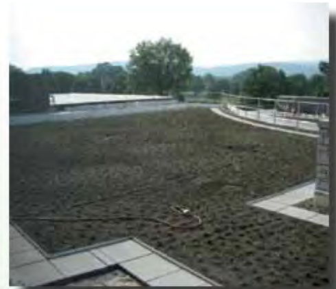
Initial Green Roof Planting
