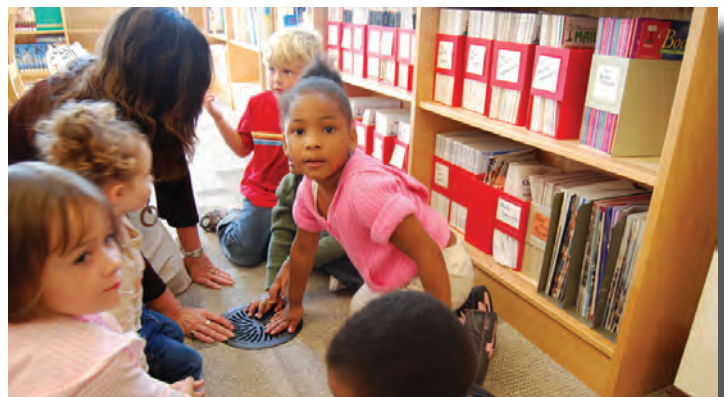
Summerfield Elementary School under floor air distribution system
