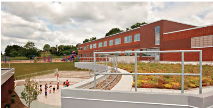
Green roof over the gymnasium lobby with an adjacent observation window for the students. Below is a courtyard utilized for several student activities
